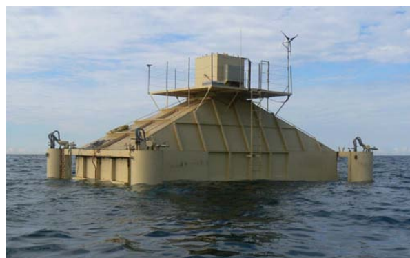
Figure 2: Second-generation Oceanlinx OWC device demonstrated in Australia.
