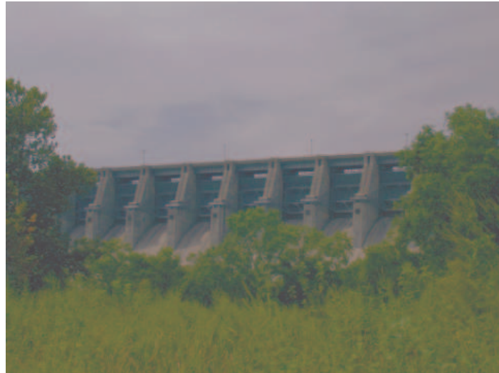
Figure 2: Typical embankment dam in Texas, USA
