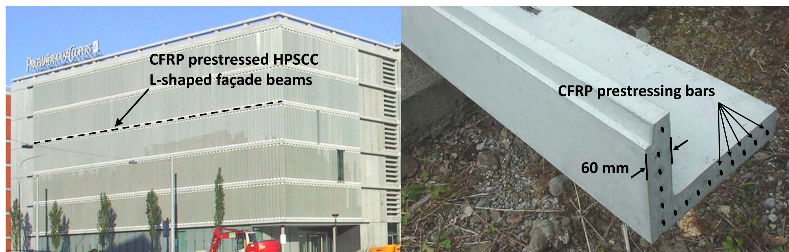
Figure 1: Application of CFRP prestressed HPSCC L-shaped beams
