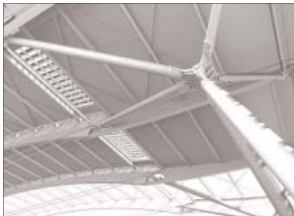
Below: Detail of T5 roof Bottom: Cross Rail tunnels will use sprayed concrete linings, allowing tunnel cross sections to be varied
